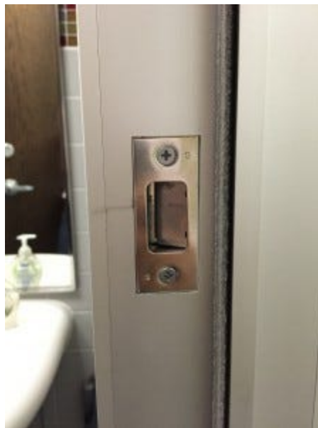
See how the pocket looks blocked by a silver panel? That's the flipper of the switch.
